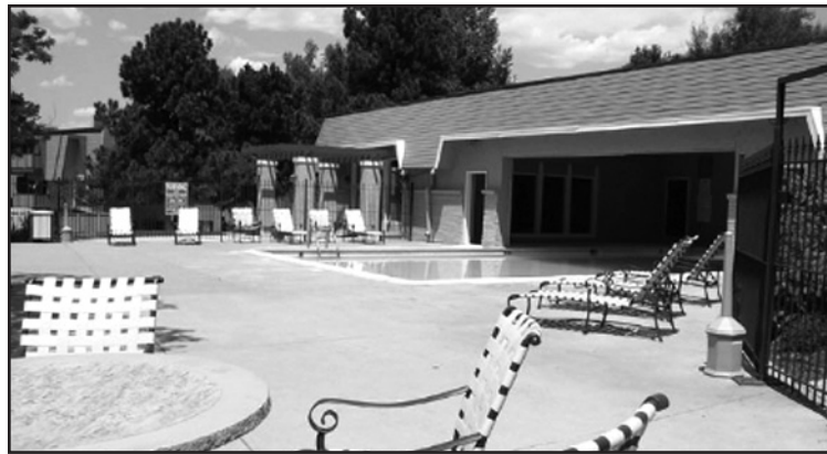
Villas at Parker faces major remediation by its new owner.
